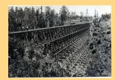
146 feet high, 82 feet wide at the base, and 12 feet wide at the top. At the time, it was one of the largest and tallest structures of its kind. The earthquake of 1906 caused the trestle to "collapse like a row of dominoes" but it was quickly rebuilt closely following the original specifications. **Click Here** to see a photo of the collapsed bridge and to read more.
